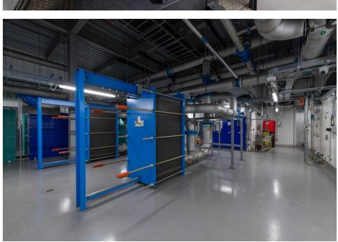
6MW of cooling water and power distribution in CR4
